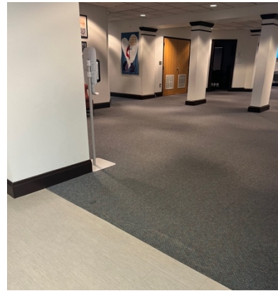
Current transition between old and new flooring in main lobby.
