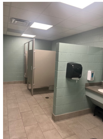
Renovations to the first floor restrooms which show planned updates to the second floor restrooms.
